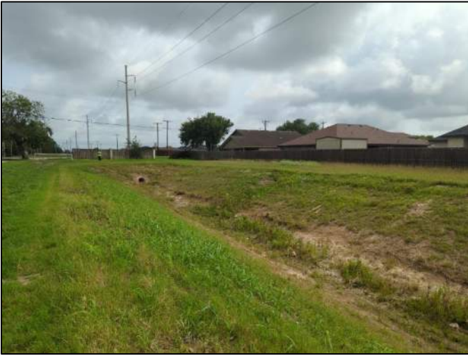
Photo 1. Existing drainage ditch south of FM 2480 (Old Port Rd), viewing northeast
