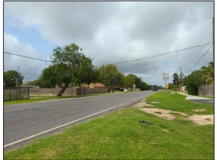
Photo 4. FM 2480 (Old Port Rd) with mowed grass roadsides, viewing southwest
