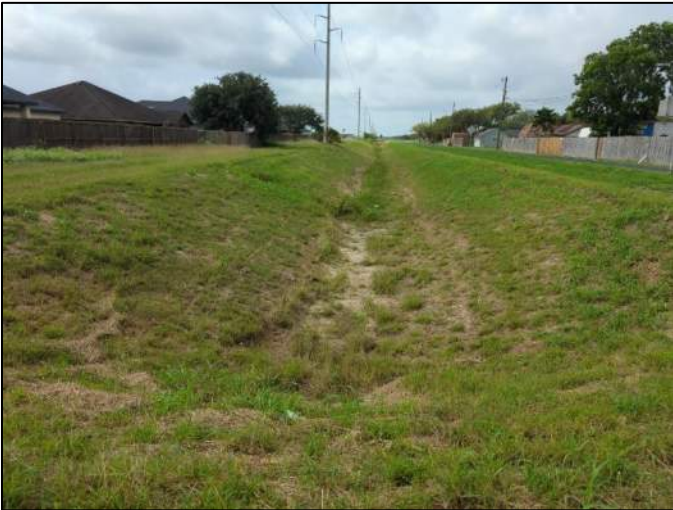
Photo 3. Existing drainage ditch south of FM 2480 (Old Port Rd), viewing south
