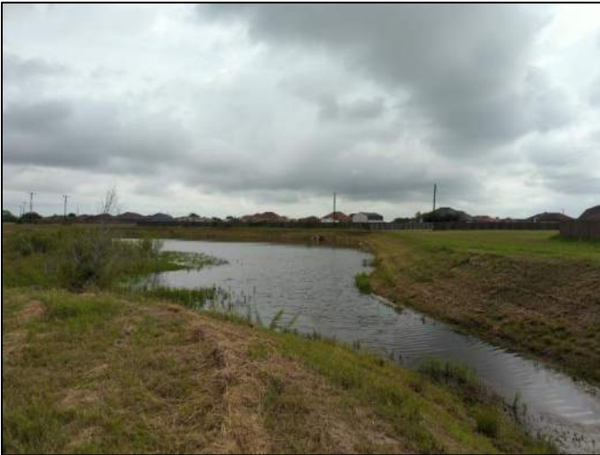
Photo 19. North end of drainage ditch with detention pond, viewing northeast
